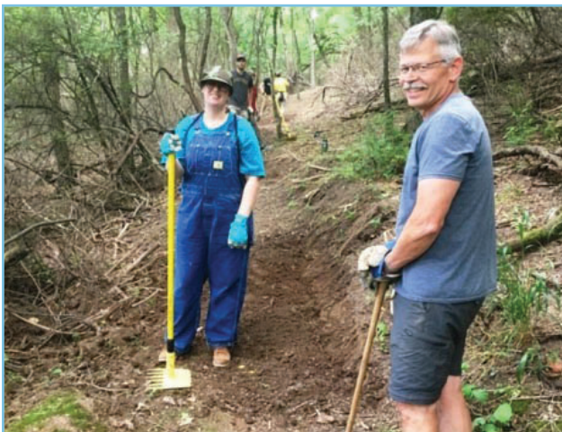
Harris Ridge Trail Construction
