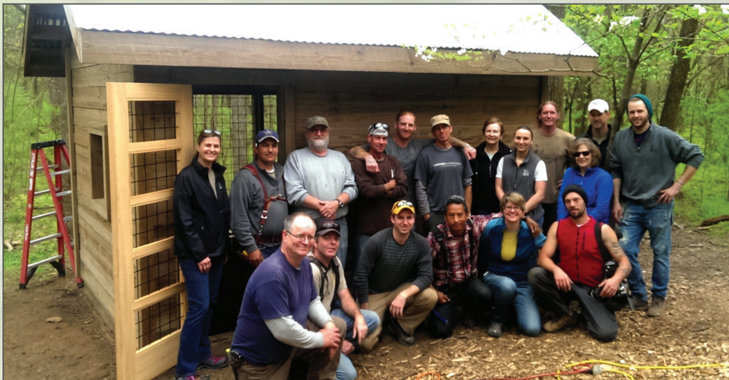
The Porch Company of Nashville rebuilds the historic Valve house at Radnor Lake for their 2016 employee community project.
